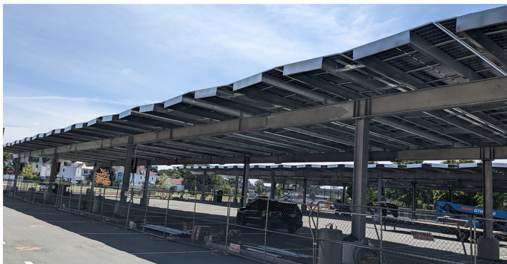
Solar canopies under construction at Beverly Middle School Aug. 16, 2022
